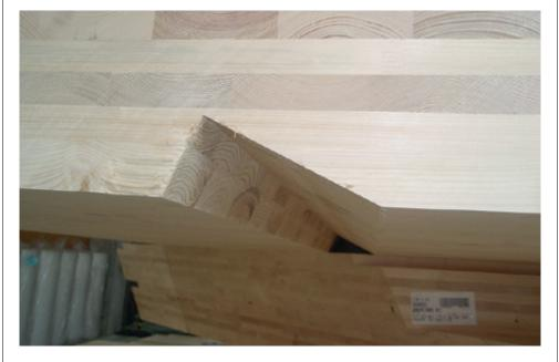
4. Rafter roof (rafter cut-outs in the CLT wall)
